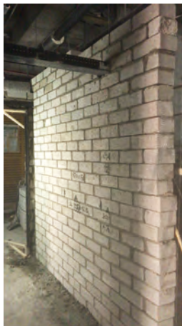
Brick laying works
