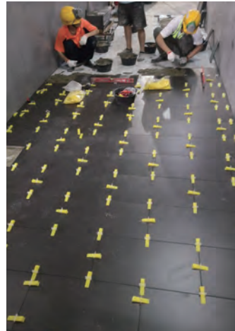
Tile laying works
